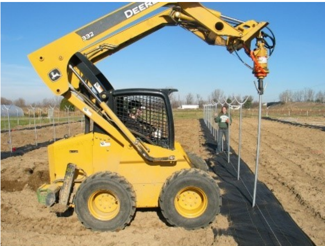
Figure 22: Multi-bay tunnels; ground posts (legs) are augered in at pre-marked positions.
