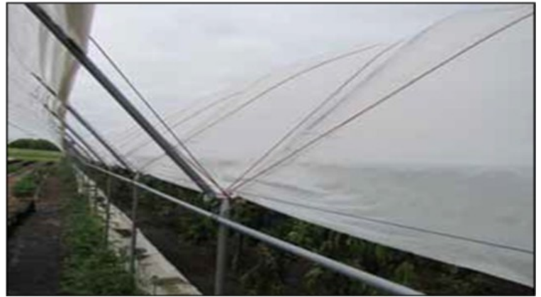
Figure 45: Multi-bay tunnels are vented by opening the plastic film covering the ends of the hoops above the side wall.
