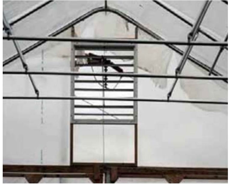
Figure 33: Vent at the peak of a gothic-style high tunnel.
