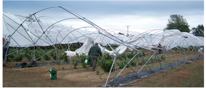
Figure 11: High wind damage to a multi-bay style tunnel.
