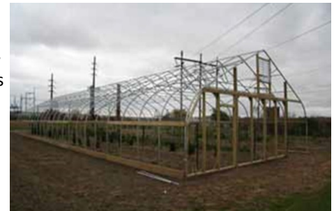
Figure 17: Peak-style (gothic arch) high tunnel framing (above)—side view showing base and hip boards and end door construction of (L to R below) door stop, pulley system for door closure, door closure.
