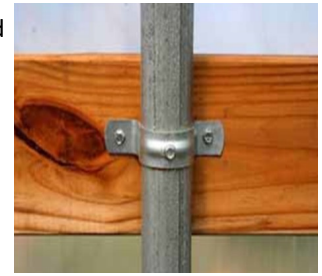
Figure 16: Fastening batten board to frame.
