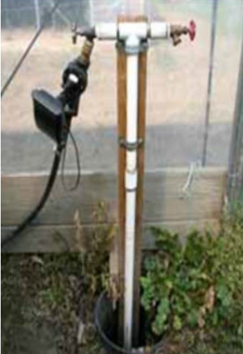
Figure 5: Water supply (vertical standpipe) to the inside of a tunnel showing (left) a faucet used for drip irrigation (with an irrigation timer directly attached to the faucet), and (right) an unused faucet for attaching an irrigation hose (not shown).
