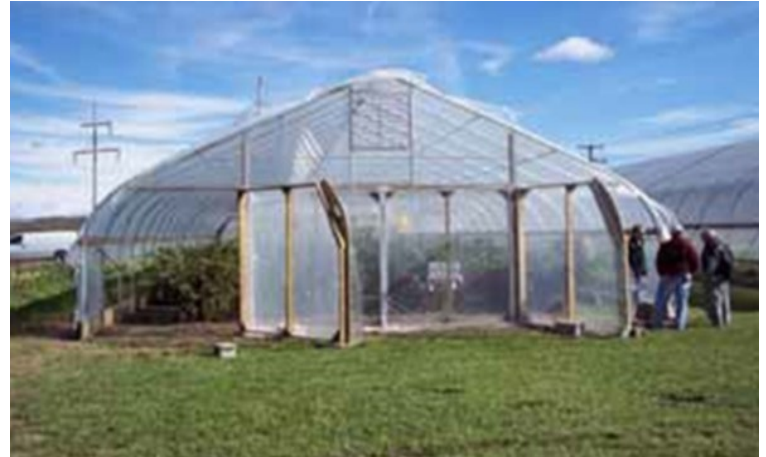
Figure 20: Hinged plastic covered tunnel doors.
